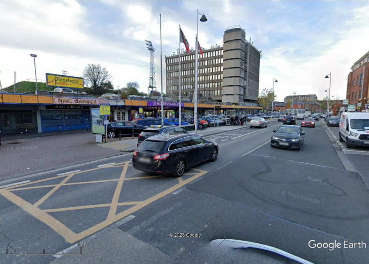
Figure 2-15: Street View of the Location looking North
